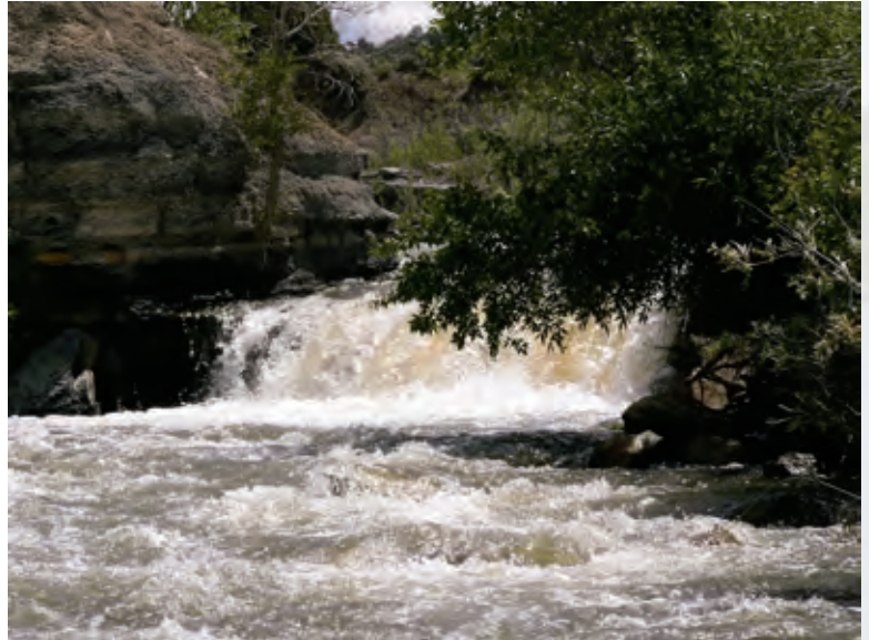
Outlet from McPhee Reservoir to Narraguinnep Reservoir
