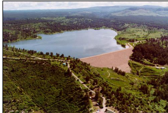
Figure 17. The Jackson Gulch Dam is an earth-fill structure standing 180 feet high with a top width of 35 feet and a length of 1900 feet.
