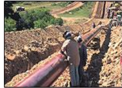
Figure 28. TransColorado Pipeline installation
